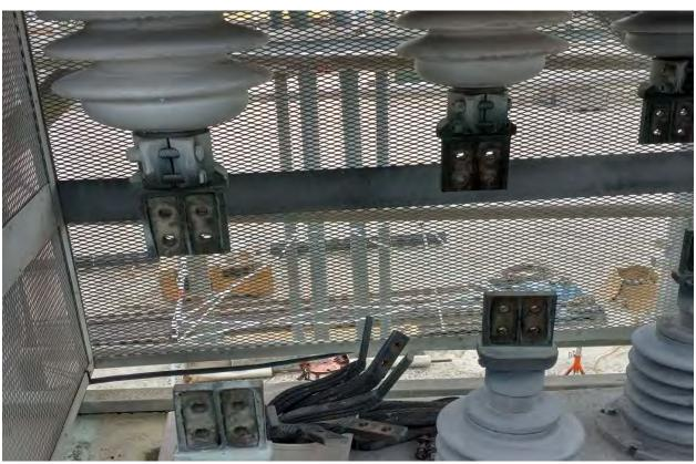
Top and Bottom Bushings at Generator and View of Eleven Inch Flex Links.
