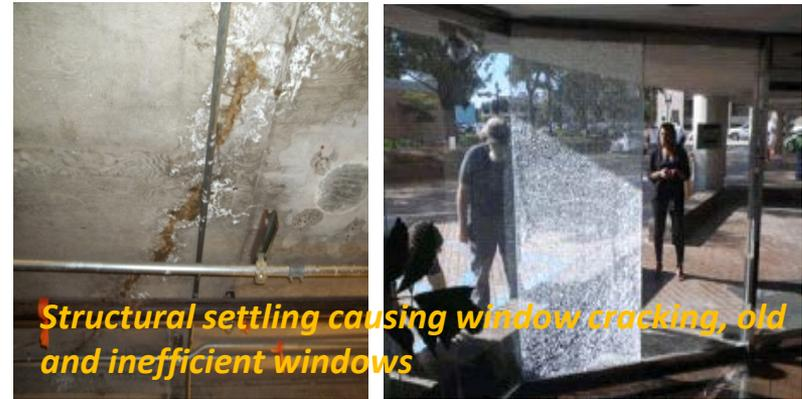
*Structural settling causing window cracking, old and inefficient windows*
